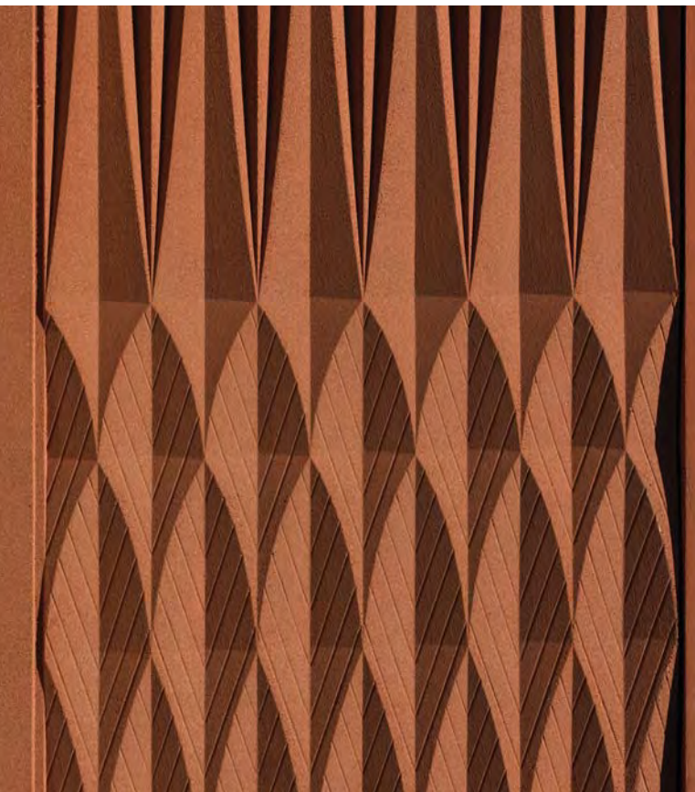
The ornmented GRC façade.
