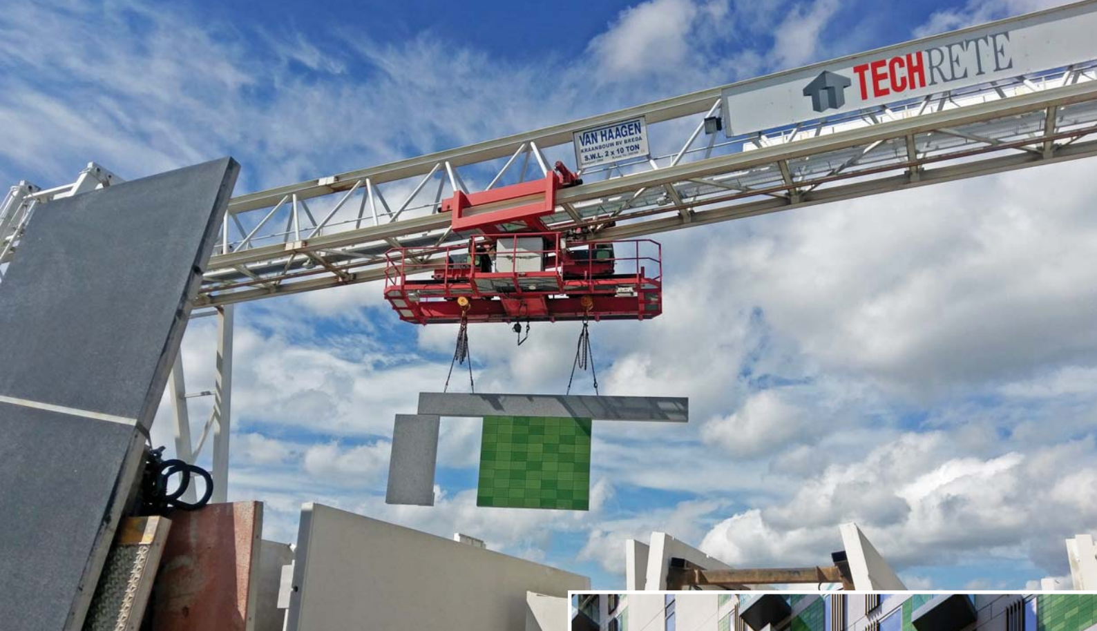
The gantry crane transports a panel across the Techrete yard.
