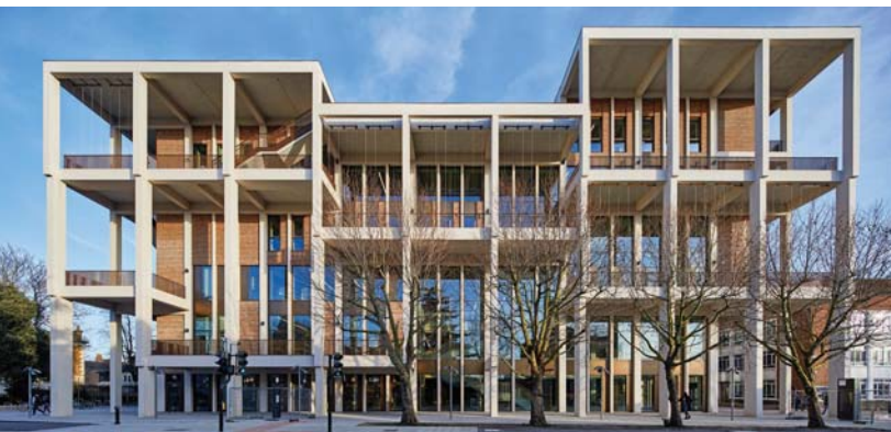
Town House, Kingston University – front elevation. (Photo: Ed Reeve.)
